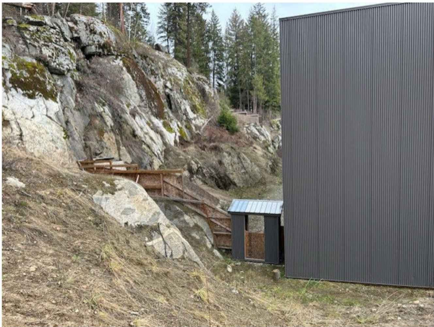
Photo 2: View toward the northeast of bedrock slope located north of site building
