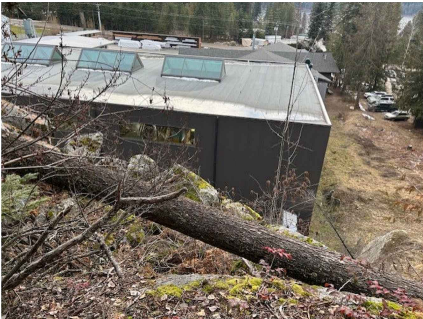
Photo 3: View toward the south from top of bedrock slope across the operational area of site
