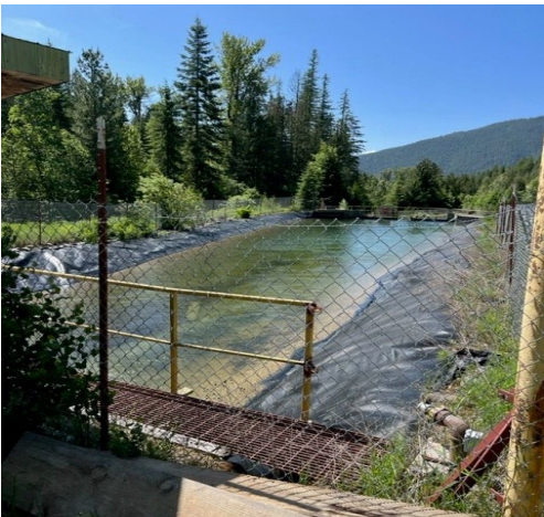
Figure 3-5 Settling Pond Arrow Water Treatment Plant
