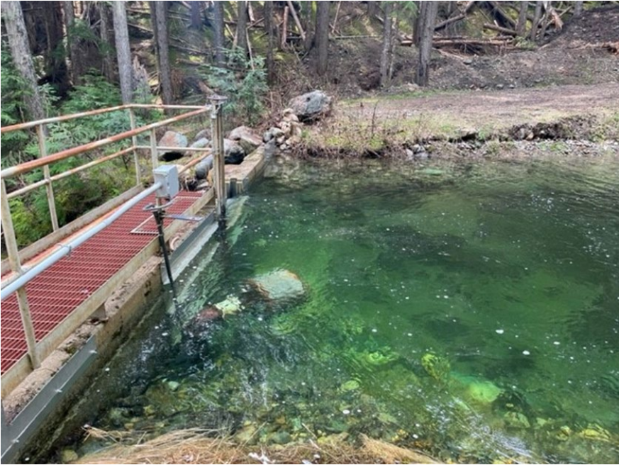
Figure 3-14 Quartz Creek Intake in Ymir
