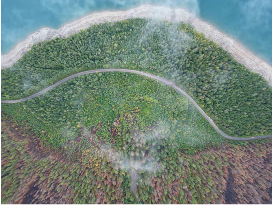
Photo 15: Lavina Creek fan with Duncan River FSR and debris flow deposit visible near apex; drone photo Oct. 1, 2024.
