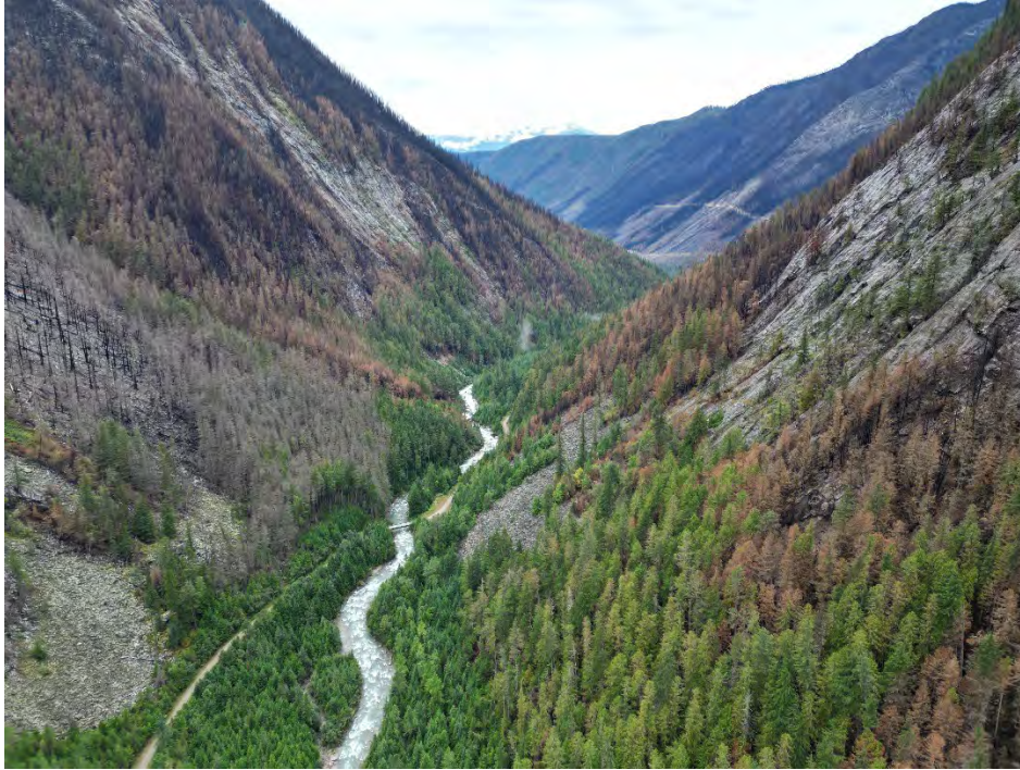
Photo 25: View downstream in Glacier Creek with Glacier Creek FSR bridge near 1000 m elevation. The bridge appears to have good clearance over a confined section of channel, reducing its vulnerability to flood events. August 28, 2024 drone photo.
