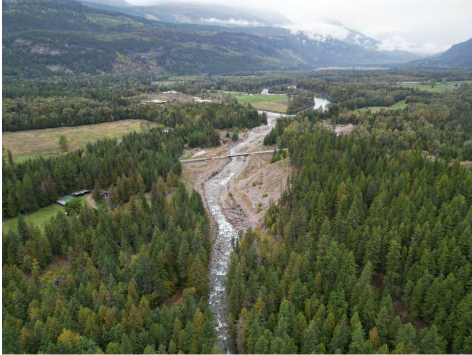
Photo 12: View downstream along Hamill Creek from near the apex of the fan. Duncan River FSR bridge and a portion of the fan is visible, along with stream training works along the creek channel which were installed in 2013 following a major flood event. Drone photo October 1, 2024.
