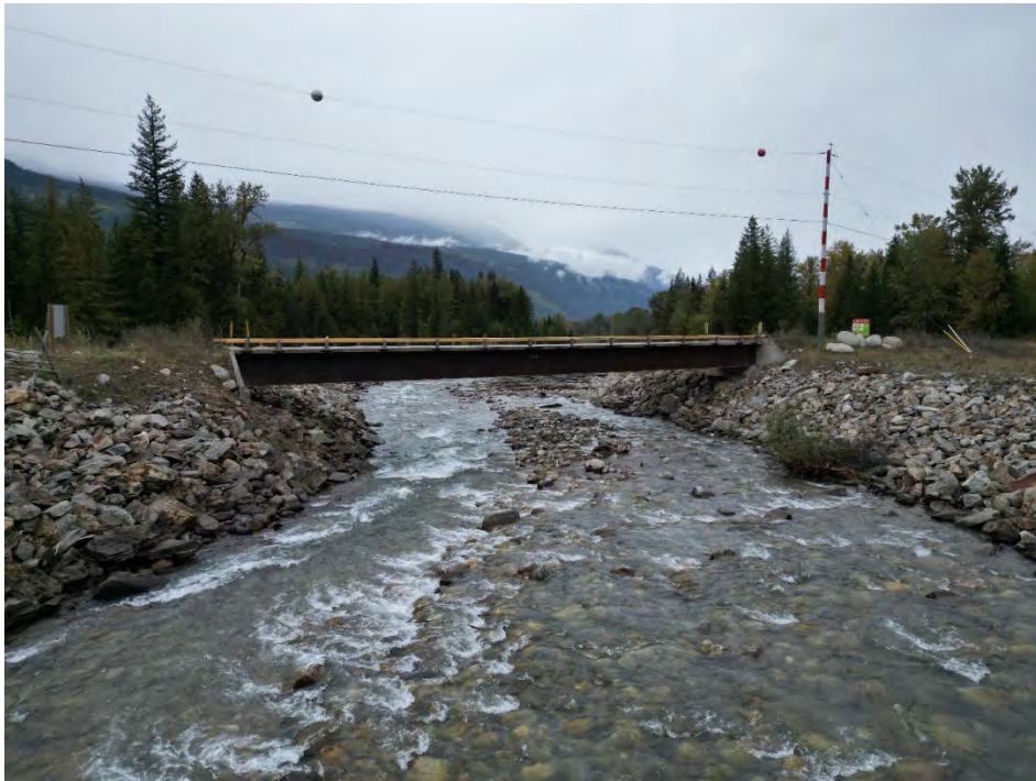
Photo 13: Hamill Creek bridge on Duncan River FSR looking downstream; drone photo October 1, 2024.
