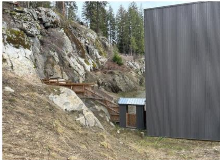
Figure 4: Photos of Bedrock Outcropping occupying approximately 15% of Lot 3 (Active Earth, 2025)
