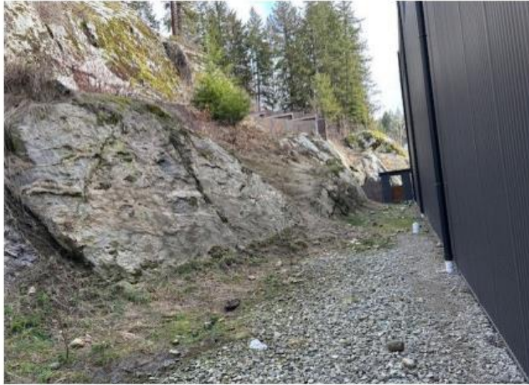
Photo 1: View toward the east of bedrock slope located adjacent and north of site building
