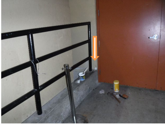
Sample 4: Plaster; west wall at north end by Zamboni exit door
