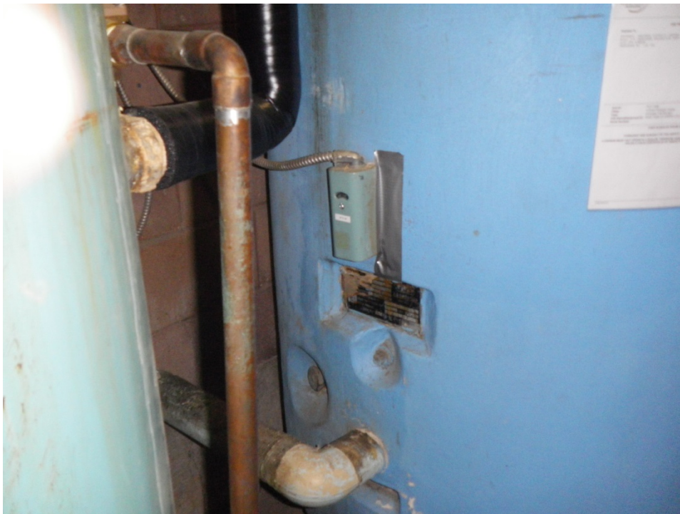
Sample 14: Mechanical room lower floor across from arena dressing rooms; tank insulation sample
