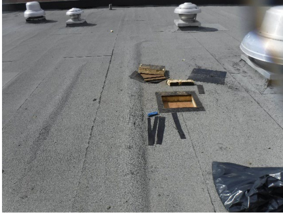
Sample 13-16: South roof bottom felt over ply (13); South roof layer above bottom felt at bottom of foam insulation (14); South roof top layer above foam insulation (15); South roof top roll on roof shingle (16)
