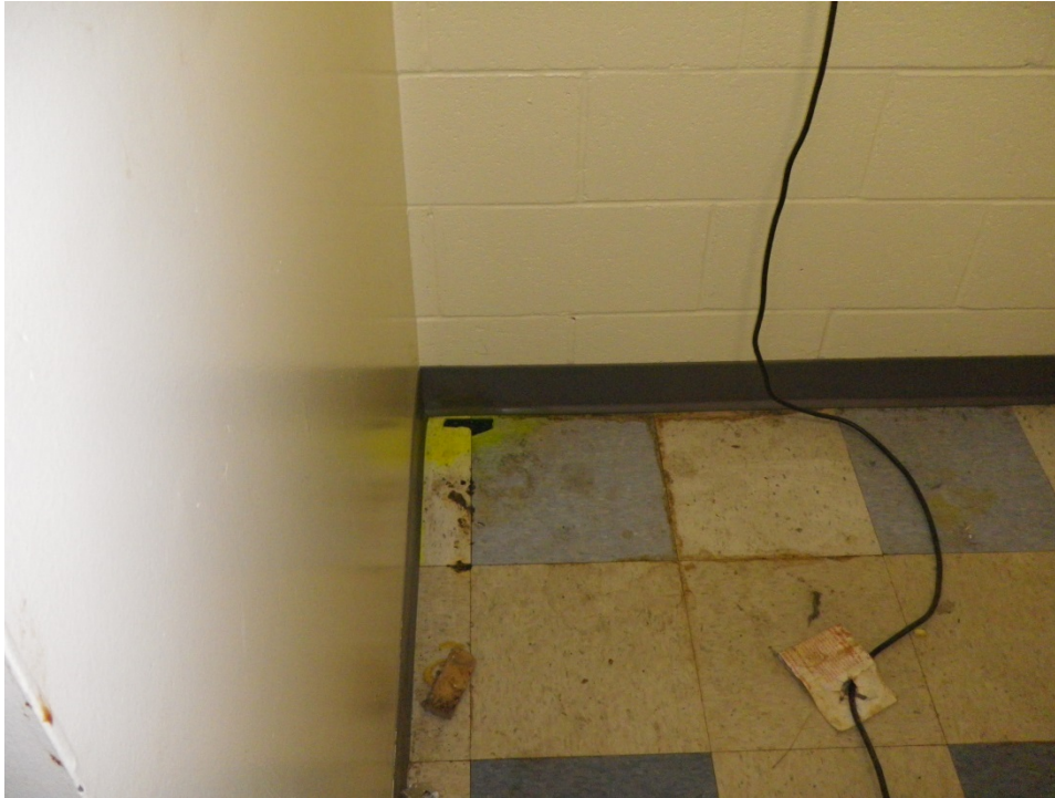
Sample 9: White vinyl floor tile in kitchen alcove behind portable fridge; includes black mastic glue
