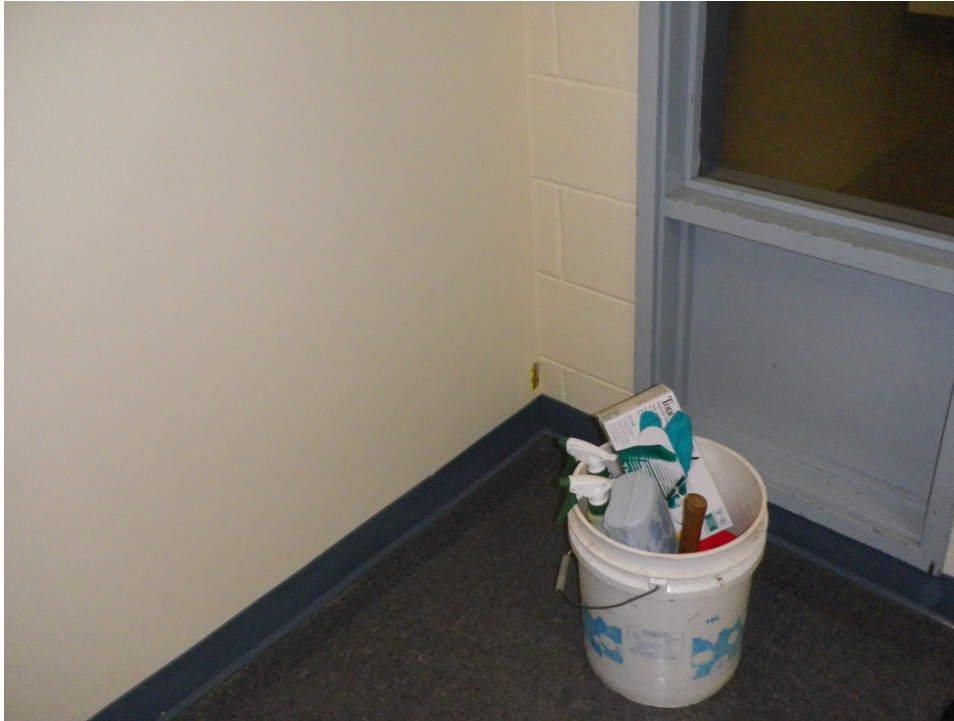
Sample 5: Drywall mud sample location, Valhalla room
