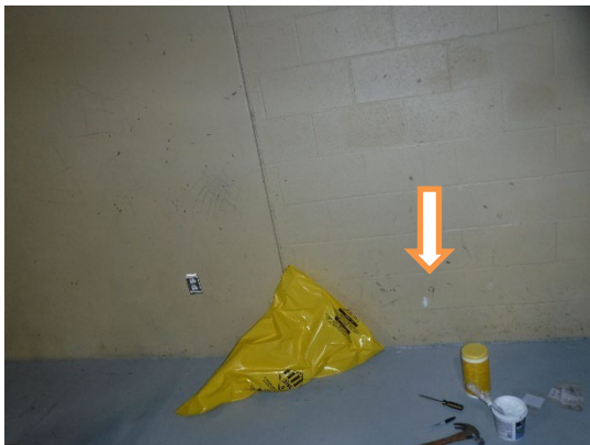
Sample 9: Mortar; west wall middle on cinderblock
