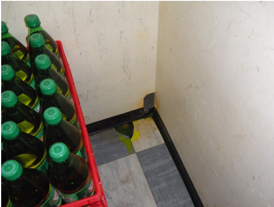
Sample 10: Greyish vinyl tile with streaks in kitchen dry good room: includes black mastic
