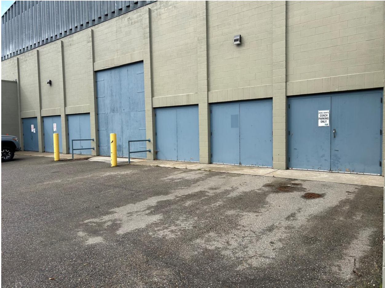
Castlegar and District Community Complex – East Elevation Arena Egress Doors 2101 6 th Ave, Castlegar, BC
