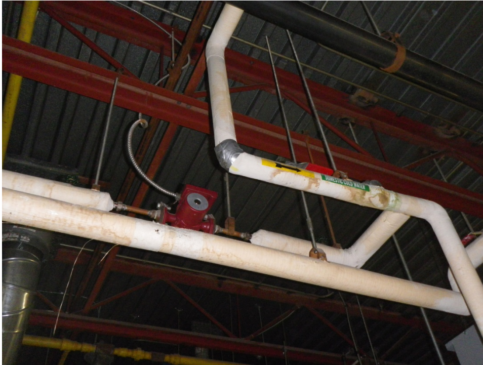
Sample 23: Pool mechanical room, pipe elbow cold water return; pipe elbow sample
