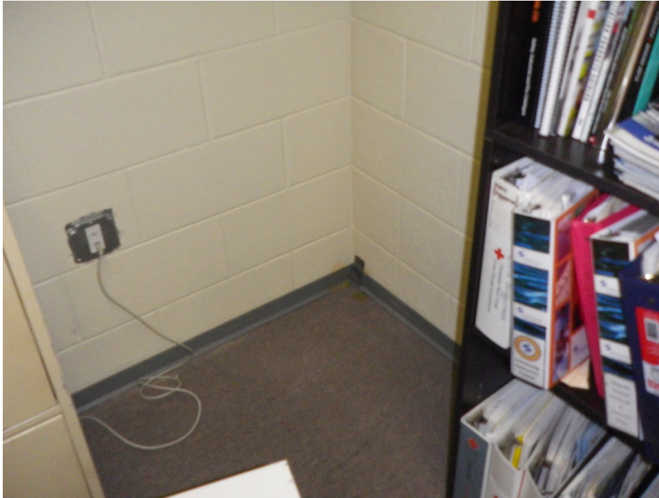
Sample 7: Gail Briggeman's office NE corner floor tile sample under rug; includes mastic
