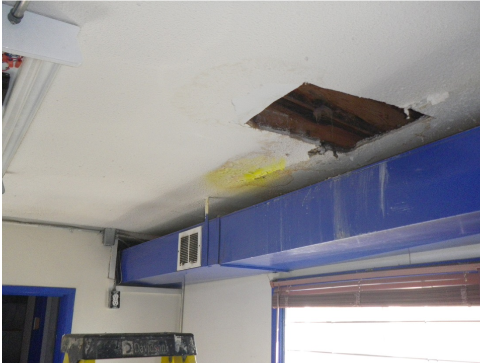
Sample 15: Old Rebels room office; ceiling texture coat sample
