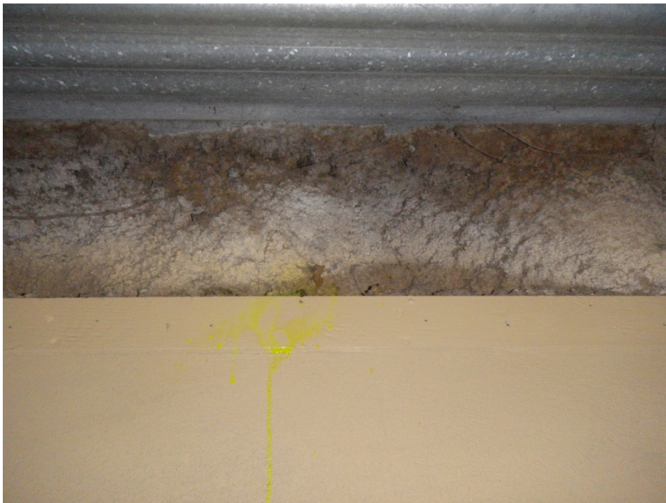
Sample 20: Arena, top of bleachers, west wall between wall and ceiling; insulation sample
