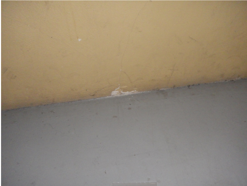
Sample 19: Arena west wall top of bleachers; stucco sample
