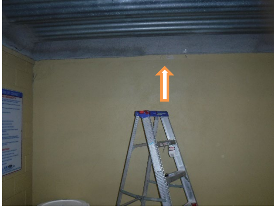
Sample A: Yellow paint; west wall south on 1"x2" board (260 ppm)
