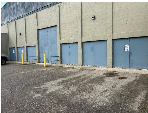
Figure 1: existing doors on east wall (photo provided by Stand)
