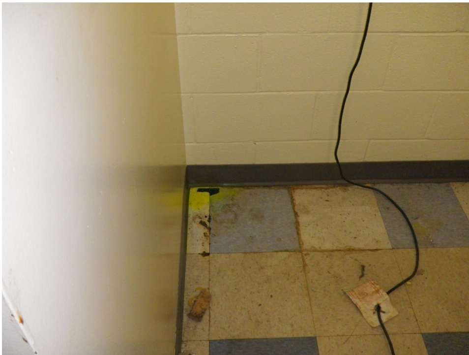
Sample 8: Light blue floor tile in kitchen alcove behind portable fridge; includes black mastic glue
