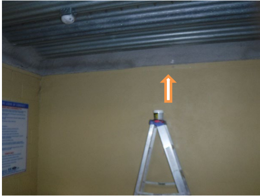
Sample 10: insulation; west wall south between wall/ceiling
