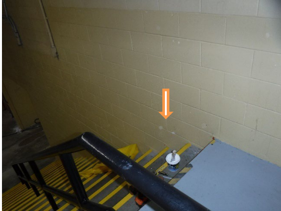
Sample 17: drilled hole, east wall south end in cinderblock (empty)
