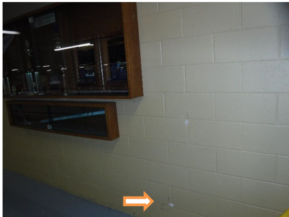
Sample 17: drilled hole in cinderblock SW corner (empty)
