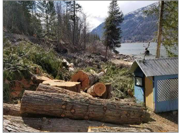
Photo 4. View of cleared trees looking west.
