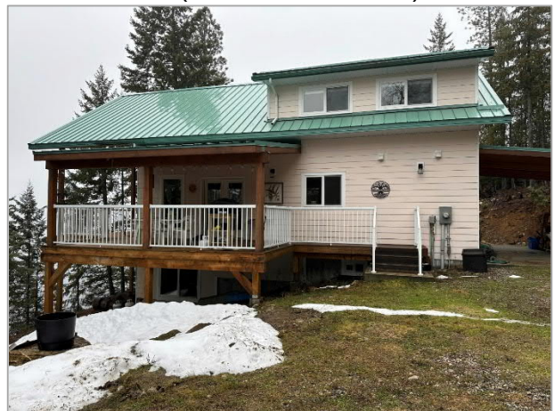
Photo 10. Existing house within 30 m riparian assessment area.
