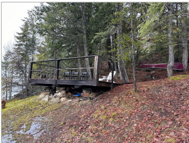
Photo 7. Existing elevated deck within 15 m setback.
