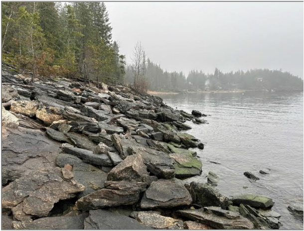
Photo 5. South view of foreshore aquatic area.
