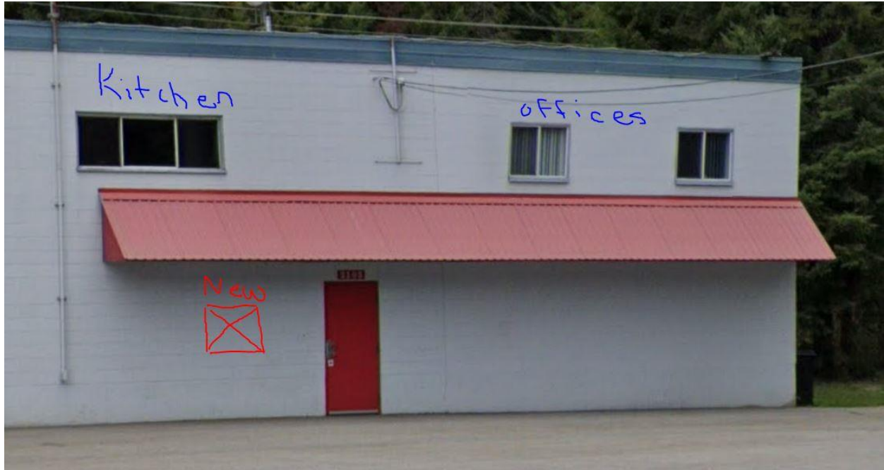
East Elevation – Windows
