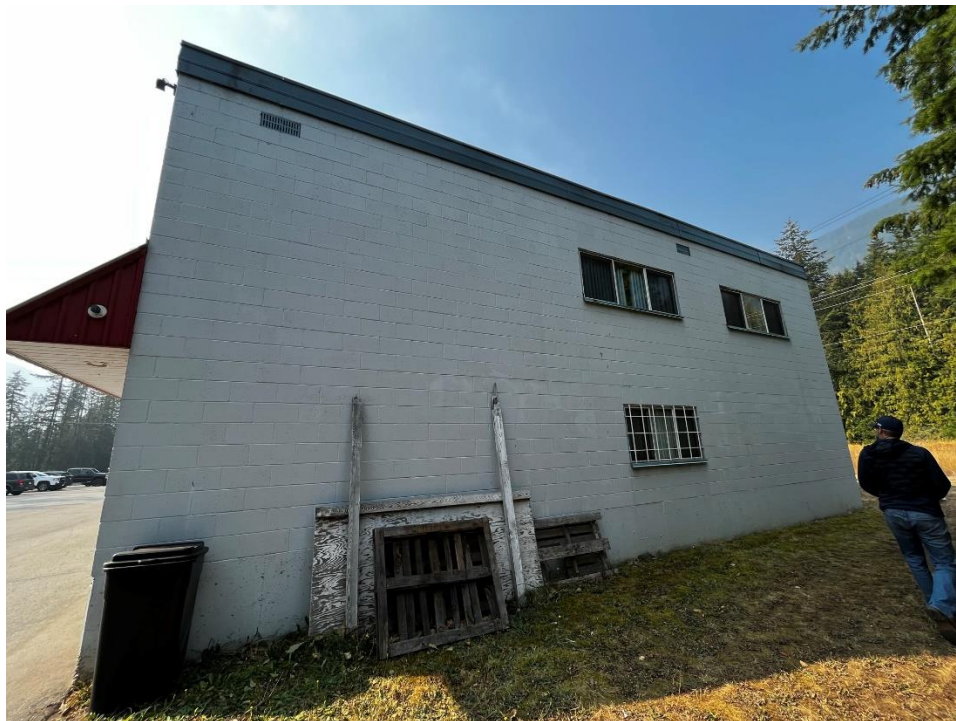
North Elevation – Windows
