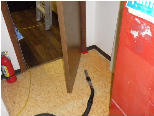
Figure 38: Sample 13, 2nd floor, kitchen, NW corner, drywall joint compound
