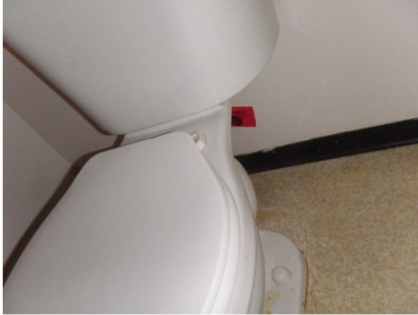
Figure 91: Sample E, 2nd floor men's washroom behind toilet east wall, beige wall paint
