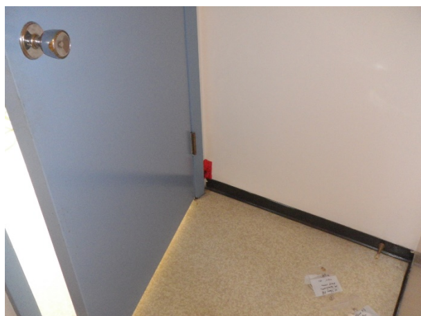
Figure 8: Sample 10; 2nd floor men's washroom SW corner, drywall joint compound
