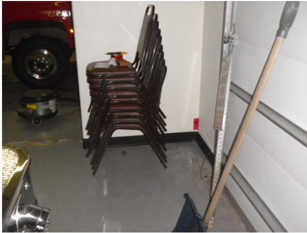
Figure 56: Sample 1, main floor main bay, NE corner, drywall joint compound
