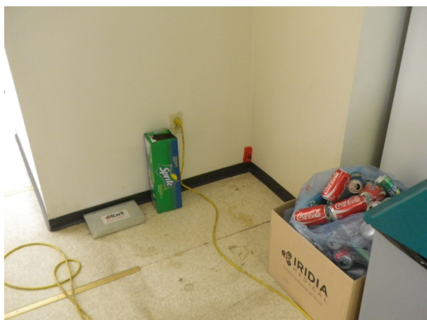
Figure 10: Sample 12, 2nd floor recreation room, SE corner, drywall joint compound
