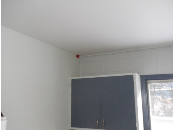
Figure 83: Sample 11, 2nd floor kitchen, NE corner drywall joint compound
