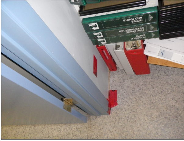
Figure 1: Sample 1, sheet vinyl flooring (grey pebble) 2nd floor training room in A/V room NE corner
