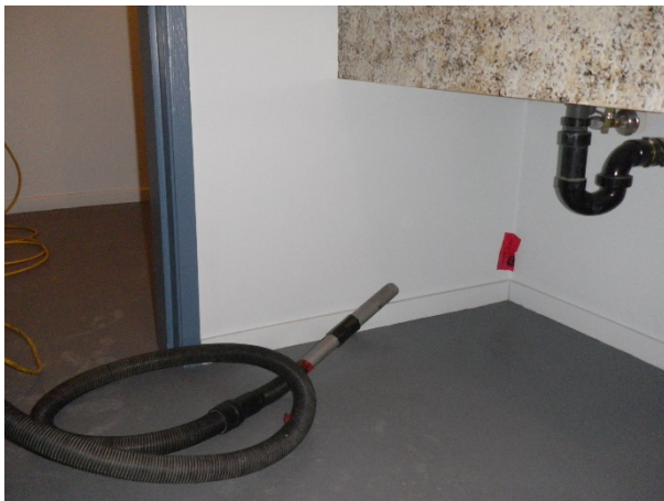
Figure 78: Sample 6, main floor north washroom SE corner drywall joint compound
