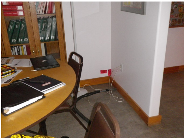
Figure 66: Sample 11, 2nd floor, recreation room, SE corner, drywall joint compound
