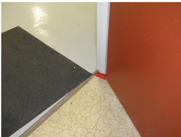
Figure 34: Sample 9, main floor hallway by north door, sheet vinyl flooring
