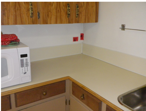
Figure 37: Sample 12, 2nd floor kitchen SE corner, drywall joint compound
