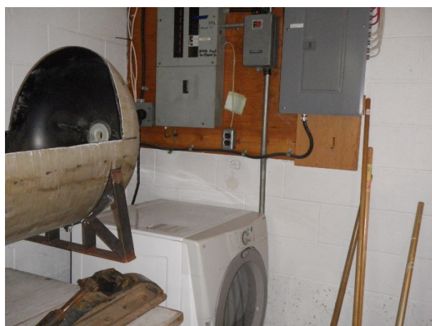
Figure 72: Sample 2, main floor workshop north wall by panel, vermiculite insulation (trace actinolite asbestos)
