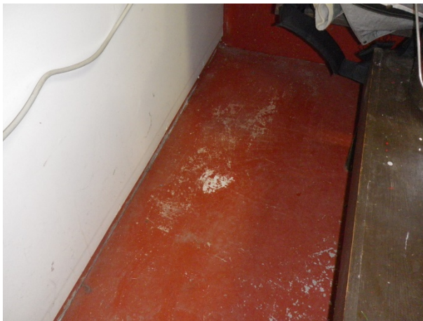
Figure 94: Sample B, main bay NW corner, red floor paint on concrete (5480 ppm)
