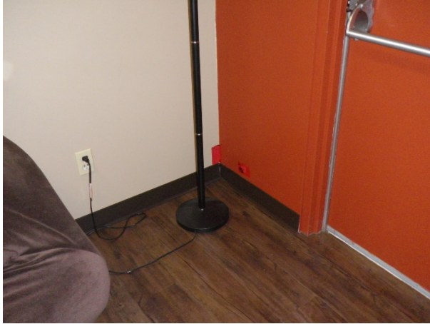
Figure 105: Sample G, 2nd floor family room, SE corner, red paint on wall
