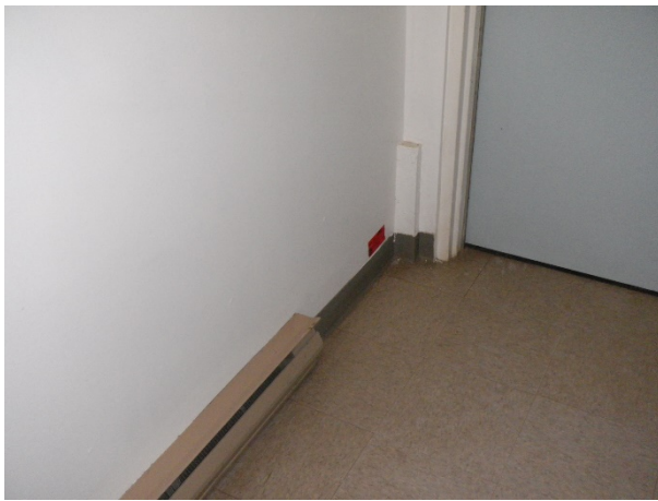
Figure 108: Sample B, main floor hallway, west wall by exit white paint on wall
