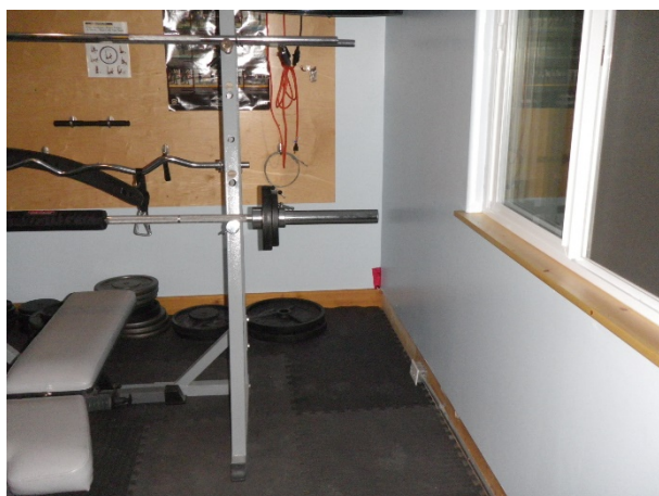
Figure 69: Sample 14, 2nd floor exercise room, SE corner drywall joint compound
