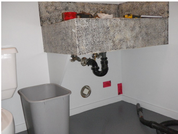
Figure 120: Sample B, main floor south washroom, north wall middle, light blue paint on wall
