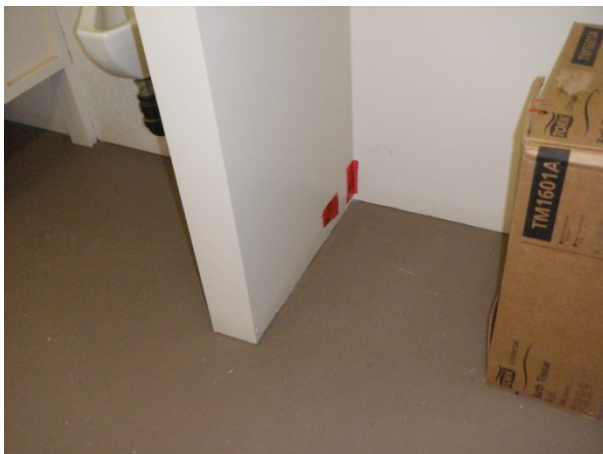
Figure 109: Sample C, main floor men's washroom south wall beige paint on wall
