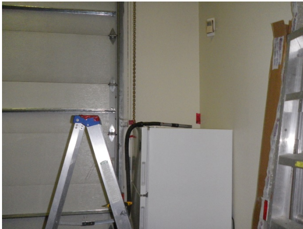
Figure 57: Sample 2, main floor main bay SE corner, drywall joint compound
