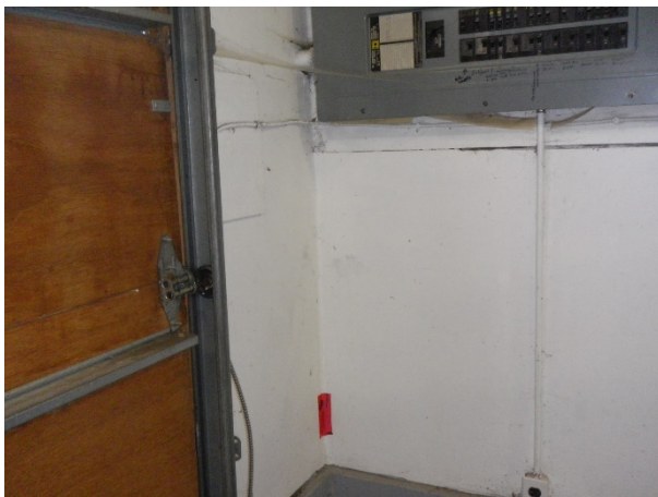
Figure 40: Sample 1, main bay SE corner, drywall joint compound
