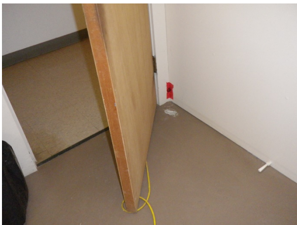
Figure 46: Sample 7, main floor, men's washroom, NE corner, drywall joint compound
