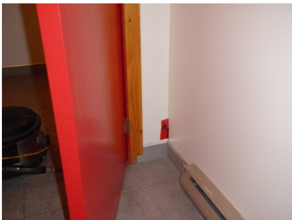
Figure 64: Sample 9, main floor men's washroom, SE corner, drywall joint compound
