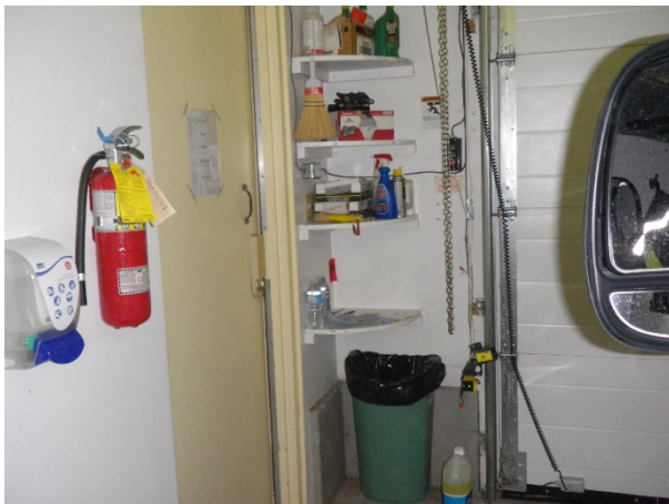
Figure 54: Sample 15, ambulance bay, NE corner, drywall joint compound
