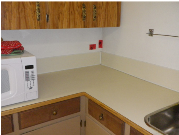
Figure 106: Sample H, 2nd floor kitchen, SE corner off white paint on wall
