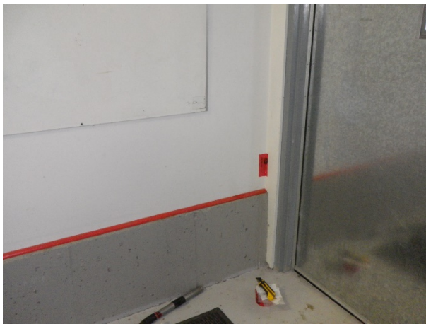
Figure 27: Sample 2 main floor, main bay NW corner, drywall joint compound
