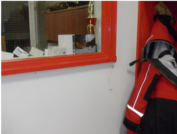
Figure 100: Sample B, main floor main bay, SW corner white paint on wall
