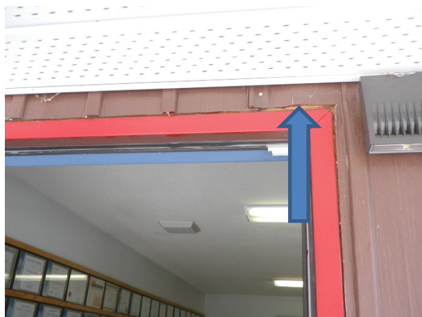
Figure 6: Sample 8, 2nd floor, NW exit, exterior above door behind siding, construction paper
