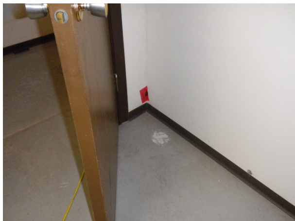
Figure 21: Sample 6, main floor men's washroom NE corner, drywall joint compound
