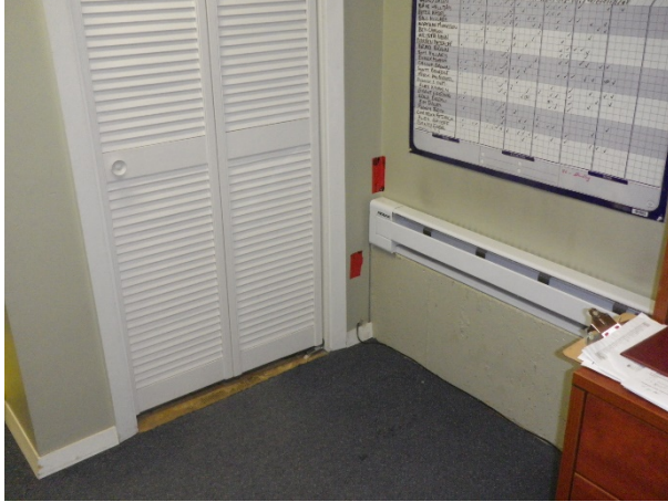
Figure 102: Sample D, main floor office, SW corner olive paint on wall
