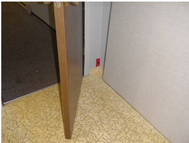
Figure 25: Sample 11, 2nd floor, kitchen NE corner, drywall joint compound
