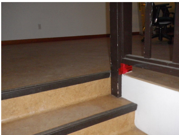
Figure 112: Sample F, 2nd floor stair handrail post, dark brown paint on wood post
