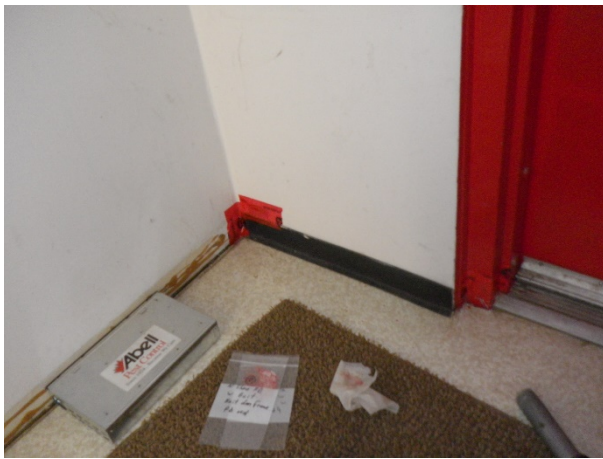
Figure 89: Sample C, 2nd floor west exit west wall white wall paint
