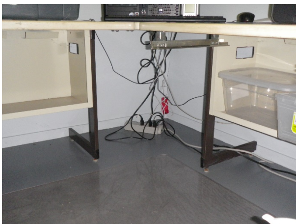
Figure 79: Sample 7, main floor office NW corner drywall joint compound
