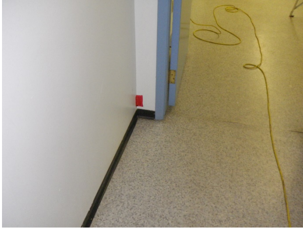
Figure 3: Sample 5; 2nd floor west hallway NW corner, drywall joint compound
