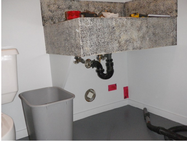
Figure 77: Sample 5, main floor south washroom, NE corner drywall joint compound
