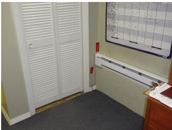
Figure 31: Sample 6, main floor office SW corner, drywall joint compound
