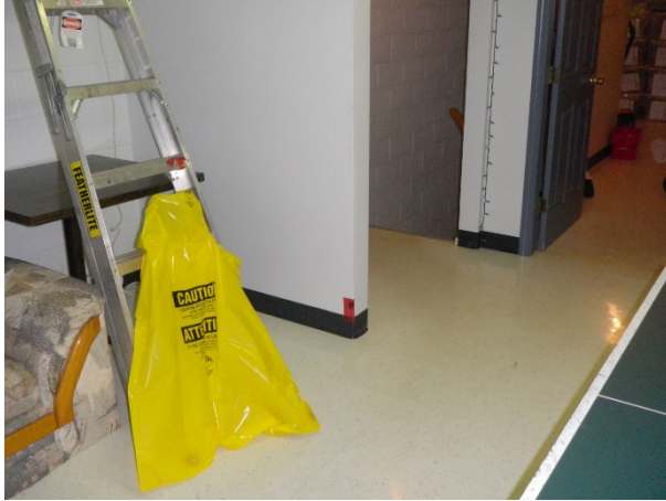
Figure 80: Sample 8, 2nd floor family room entry corner, drywall joint compound
