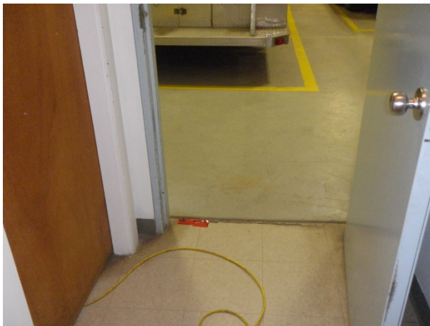
Figure 45: Sample 6, main floor hallway by east entry, vinyl floor tile
