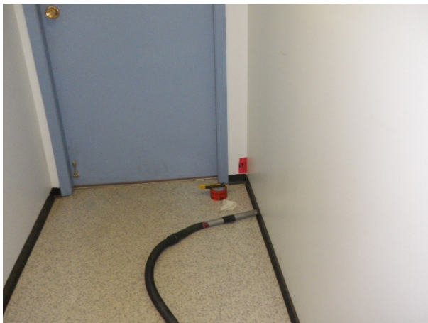
Figure 4: Sample 6; 2nd floor west hallway, SW corner, drywall joint compound
