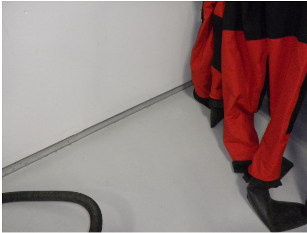
Figure 99: Sample A, main floor main bay, SW corner grey floor paint on concrete
