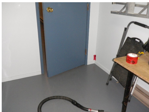
Figure 74: Sample 4, main floor workshop, SE corner drywall joint compound
