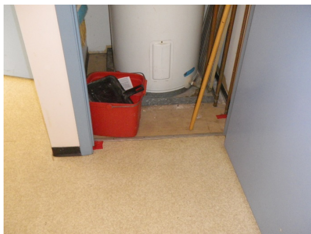
Figure 7: Sample 9; second floor men's washroom hot water tank storage room, west side, vinyl floor tile, beige 1'x1' (1% chrysotile asbestos)
