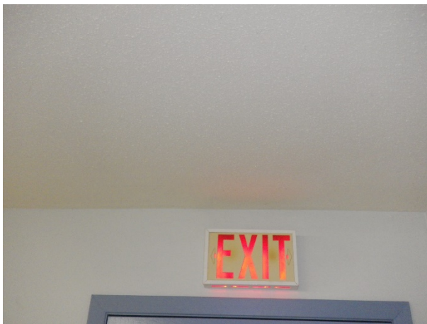
Figure 2: Sample 4; 2nd floor training room above south entry door, texture coat
