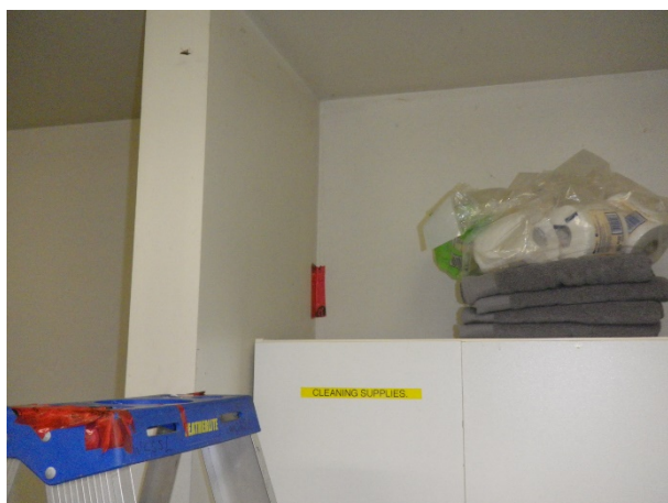
Figure 22: Sample 7, main floor men's washroom, south wall, drywall joint compound
