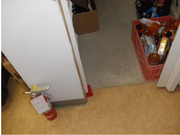
Figure 44: Sample 5, main floor office, NW corner, sheet vinyl flooring
