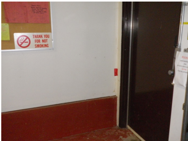
Figure 17: Sample 2, main floor main bay NE corner, drywall joint compound
