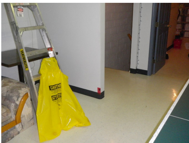
Figure 118: Sample E, 2nd floor recreation room, SE corner, white paint on wall
