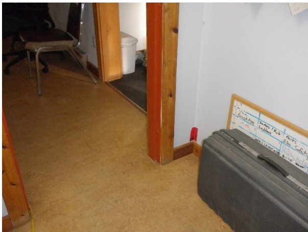
Figure 51: Sample 12, 2nd floor kitchen, NE corner, drywall joint compound
