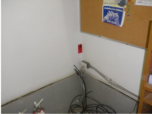
Figure 53: Sample 14, ambulance bay, NW corner, drywall joint compound
