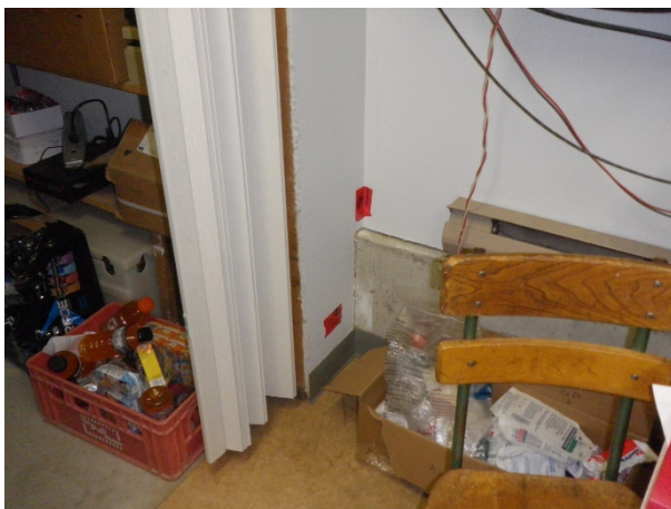
Figure 43: Sample 4, main floor office, NW corner, drywall joint compound
