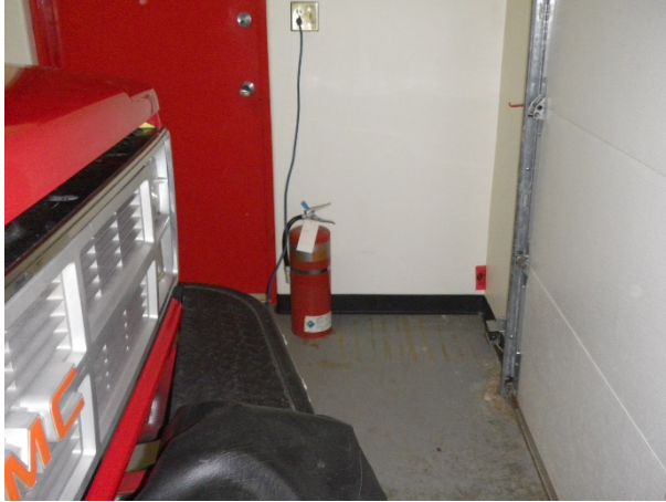
Figure 59: Sample 4, main floor, small bay NE corner, drywall joint compound
