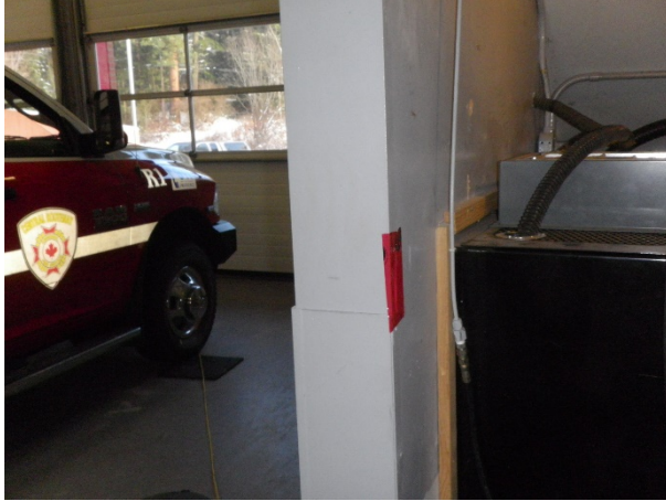
Figure 12: Sample 14, main floor south wall corner by compressor, drywall joint compound
