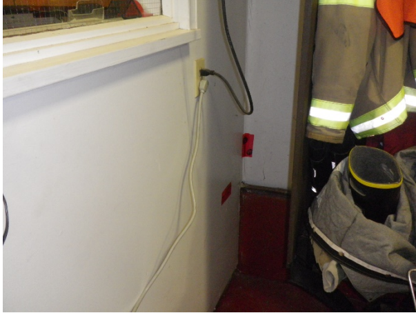
Figure 18: Sample 3, main floor main bay, NW corner, drywall joint compound
