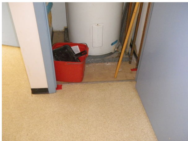
Figure 9: Sample 11, 2nd floor men's washroom at storage room by door, sheet vinyl flooring, beige pebble pattern (40% chrysotile asbestos)
