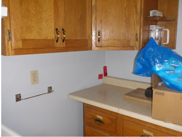
Figure 113: Sample G, 2nd floor kitchen, SW corner light blue paint on wall
