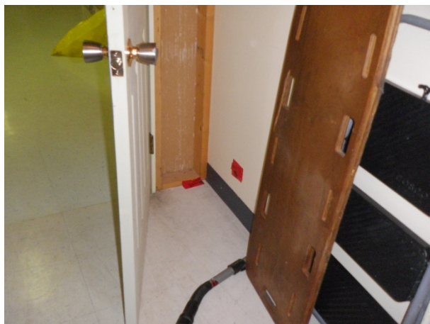
Figure 122: Sample D, 2nd floor storage room, NW corner at door, beige paint on wall
