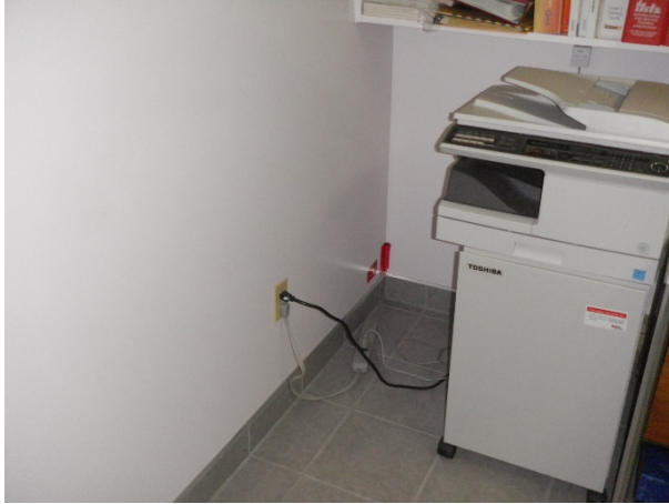
Figure 116: Sample C, main floor office, NE corner pink paint on wall
