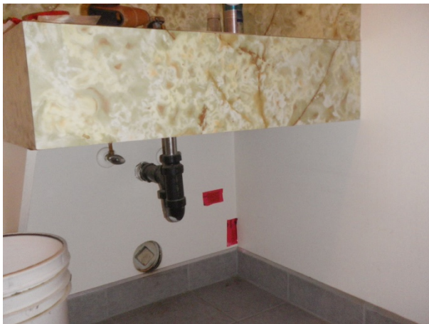
Figure 117: Sample D, main floor men's washroom, NE corner wall, white paint on wall
